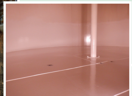
Interior Wall After
