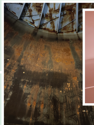
Interior Wall Before
